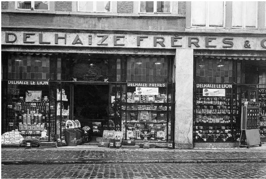
FIGURE 2 | Branch in the Rue de l'Ange, Namur, renovated in 1928 | © Archives Delhaize Group
